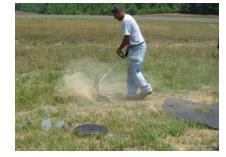
**Mat Placement: Can Mounted:** The 12 inch center hole is designed to fit snuggly around the can lid, while still allowing access to the bolts to remove the lid for general maintenance and troubleshooting of the light. Lay the mat over the light with the points of the football mat pointing in the direction lawn mower equipment will travel.
