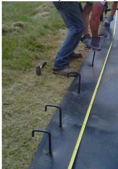
inch drill bit. You may use the top of an anchor to set your spacing from the edge of the mat. Drill through the mat and into the ground the full 6 inches. This makes a good pilot hole for the anchor. Typically the anchor can then be forced through the mat into the ground 6 inches and then driven the rest of the way with a 6-8 pound hammer.
