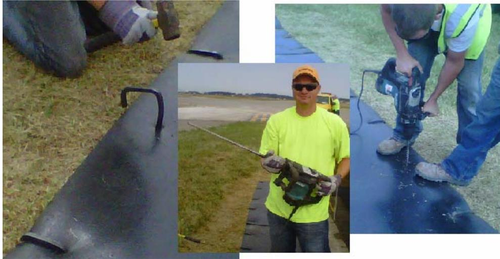
**Tools:** A line trimmer and blower for prep work where needed. A tape measure, razor knife, drill for starting anchors, A hammer drill for occasional trouble spot. And a hefty hand sledge is best for the stake anchors. Caulking gun and asphalt sealant (not provided). And Bring a Camera.\*
