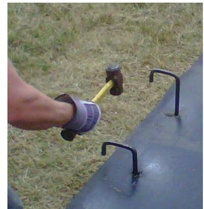
Then hammer the anchor through the pilot hole with its 2 inch pin reaching over the mats edge into the ground. The anchor is generally strong enough to penetrate rocks and buried concrete splattering.
