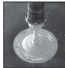
Football mat with collar insert and spiral ground anchors shown. Spiral ground anchors are secured with a 1/2-inch socket drive.
